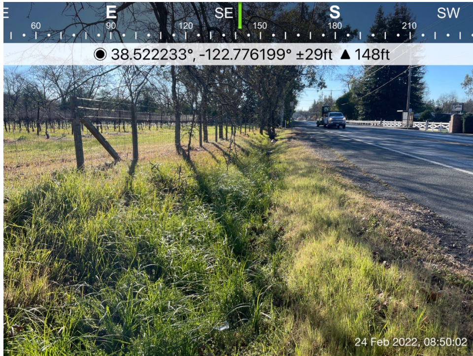
Photograph 14: Photo shows an overview of the southern roadside drainage ditch RD-02.
