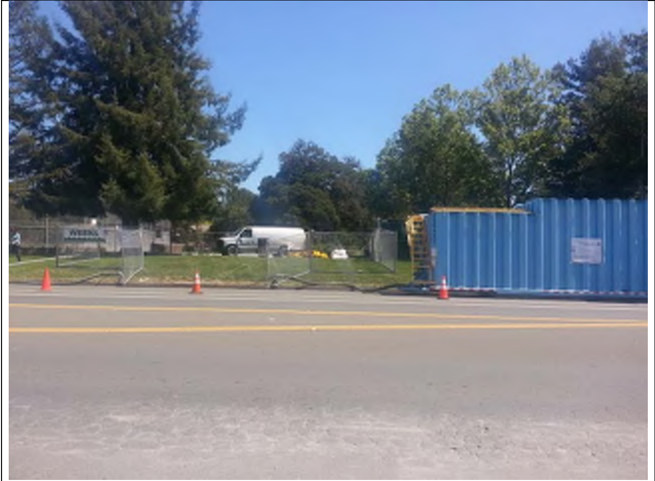
Video service at Esposti Supply Well prior to well development.
