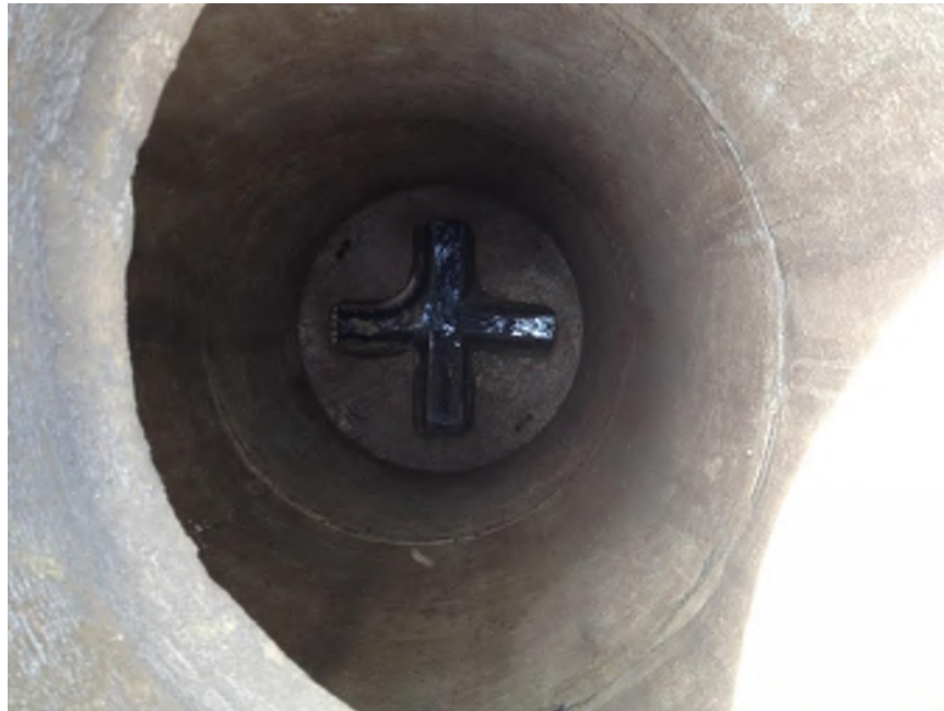
S130B Looking Inside, 12-ft from rim to bottom, 8-inch sewer
